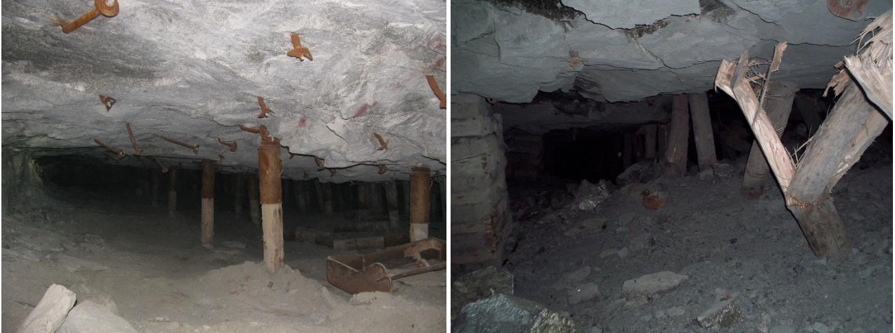
Figure S1. Photograph of a typical tabular platinum stope (left) and the hanging wall unravelling along the joints prior to a large panel collapse (right). There are many interacting blocks in the hanging wall. Note the evidence of significant closure and the broken elongates.
