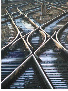
Fig. 6: Double slip switch at Munich Central Station by Láczy [39] published under a CC BY-SA 2.0 license
