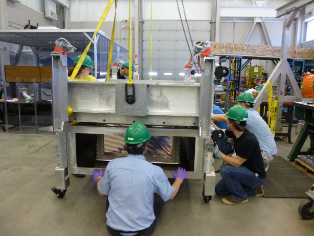
Figure 12: Motion chassis attached to enclosure and allowing the TPC to be supported and rotated.
