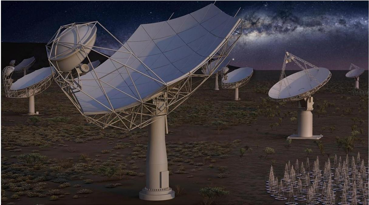
**Figure 1.** An artist vision of the SKA Core site, with some of the projected 3000 15-meter parabolic dishes and low frequency dipoles. From <http://www.skatelescope.org>.
